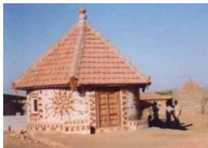
Figure 11: Stabilized Compressed earth blocks Bhunga
