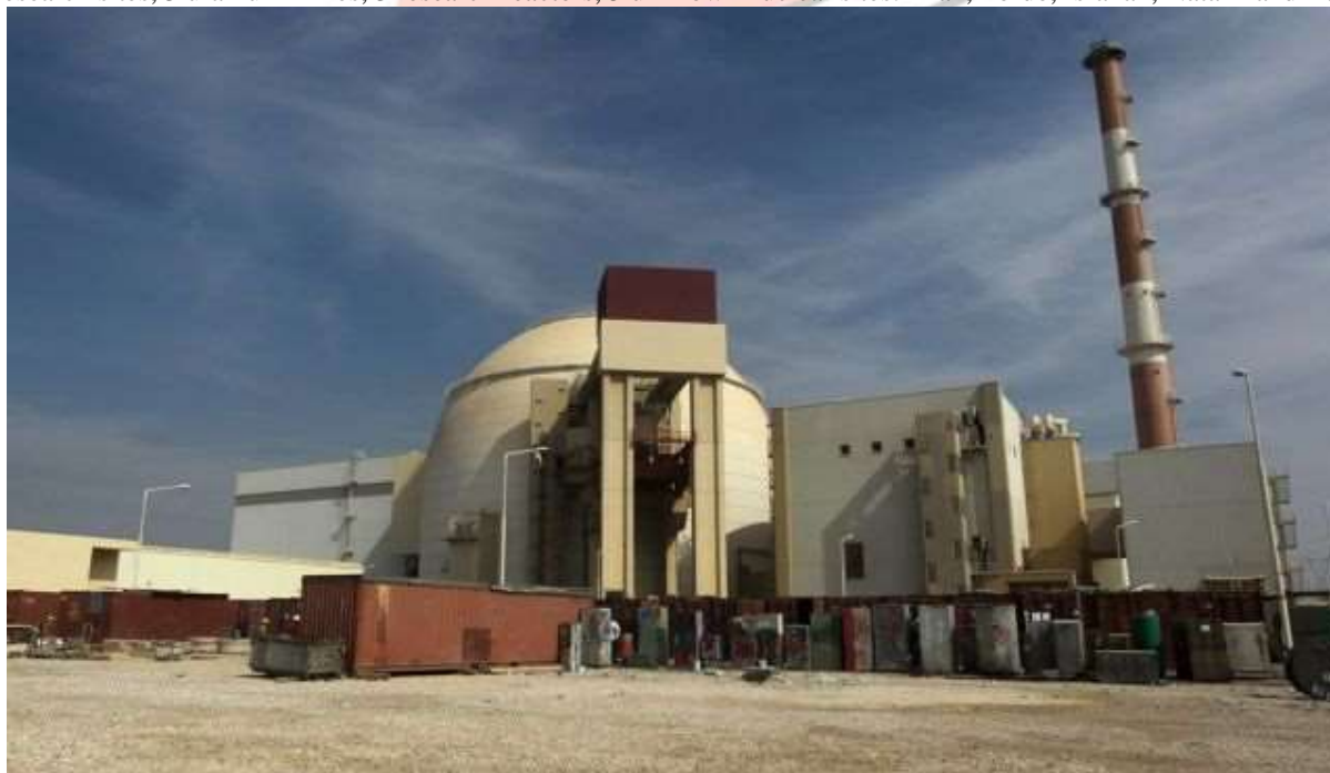
[Figure 1: Bushehr Nuclear Plant]
