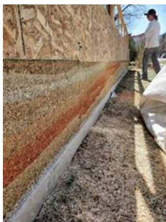
Fig.3.In-situ layered hempcrete wall construction.
